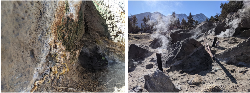
Fig. 13 A Vent Under a Rock (Left) and Capped Vents (Right) at Basalt Fumarole, Inyo National Forest, CA
